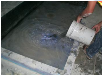
The entire pan gets flood tested.
