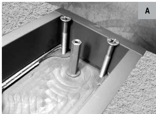
Installation of stand-off pins into end of Linear Drain base. Installation of Tile Top Strainer pins into stand-offs.
