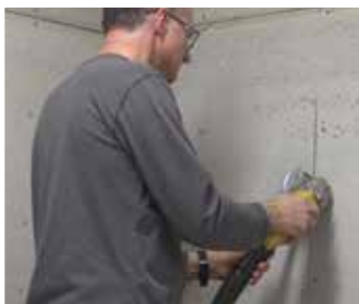
Mark and cut area for Niche
