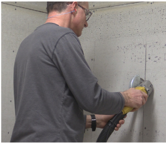
Mark and cut area for Niche
