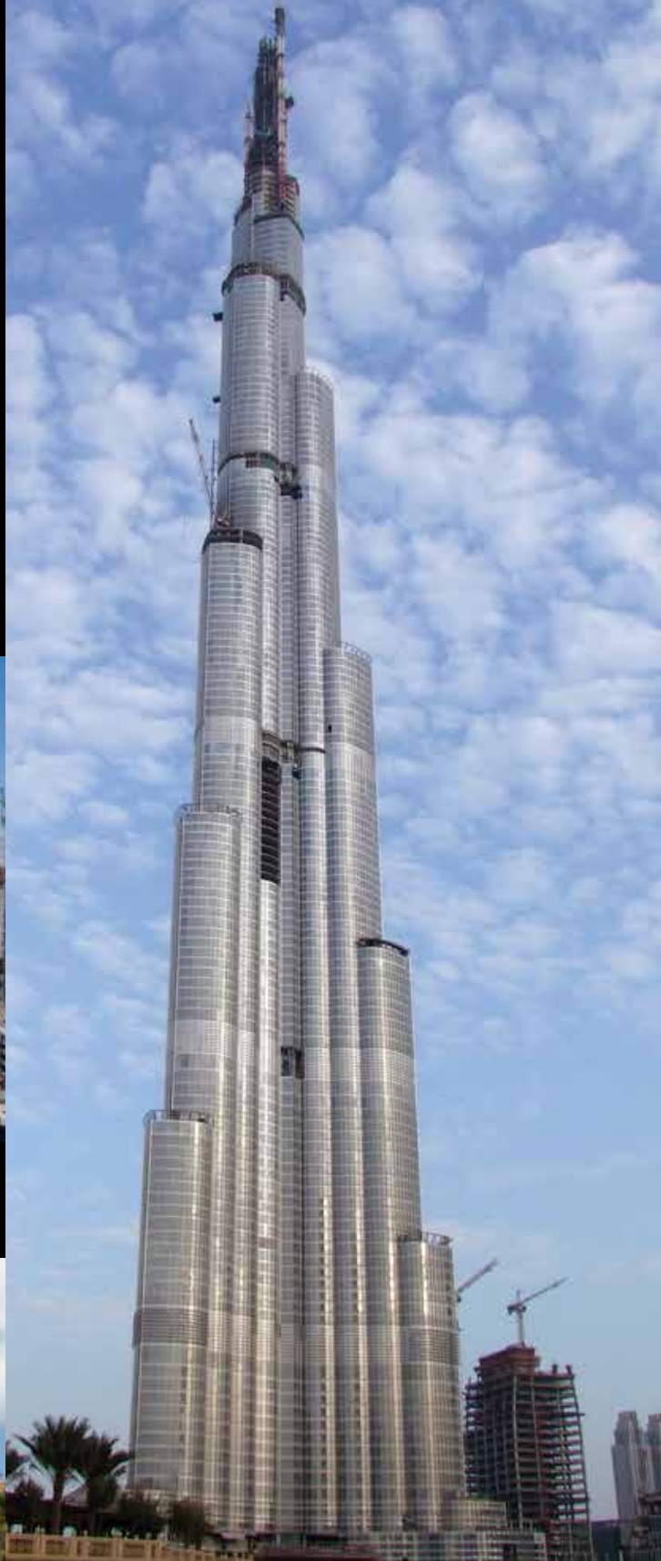
Burj Khalifa, Dubai, United Arab Emirates (UAE) Products Installed: NobleSeal TS and Chloraloy
