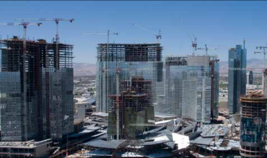
City Center Project, Las Vegas, Nevada Products Installed: NobleSeal TS, NobleBond EXT, NobleSealant 150, Shower Accessories, Noble Deck, and NobleSeal SIS
