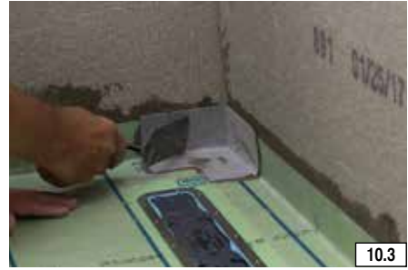
FIGURE 2: MEASURE AND CUT CURB WATERPROOFING
