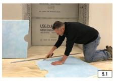
**6.2 INSTALL BASE:** Apply modified thin-set using a 1/4" x 3/8" x 1/4" square-notched trowel over the substrate and upturns. Key-in modified thin-set to the bottom and ends of the bases. Embed bases into the thin-set with slope towards drain using firm foot pressure to ensure 100% coverage and no voids.
