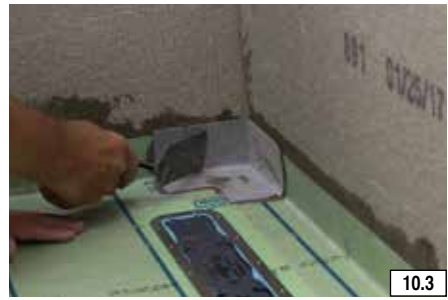
FIGURE 2: MEASURE AND CUT CURB WATERPROOFING
