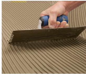
Apply thin-set to substrate
