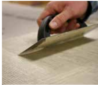
Apply thin-set to substrate
