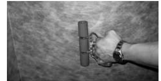
Use rubber hand roller or flat side of trowel with heavy pressure.
