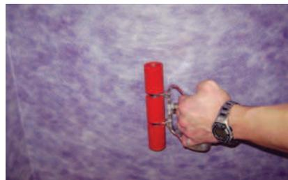
2. Embed Wall Seal with hand roller or straight edge.
