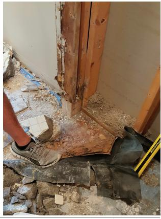
mold issues. The images scattered throughout this article, courtesy of Charles Nolen, Millers Flooring America, Lafayette, Ind., show the kinds of failures that result when low permeation waterproofing membranes are not included in steam and wet-area installations.
