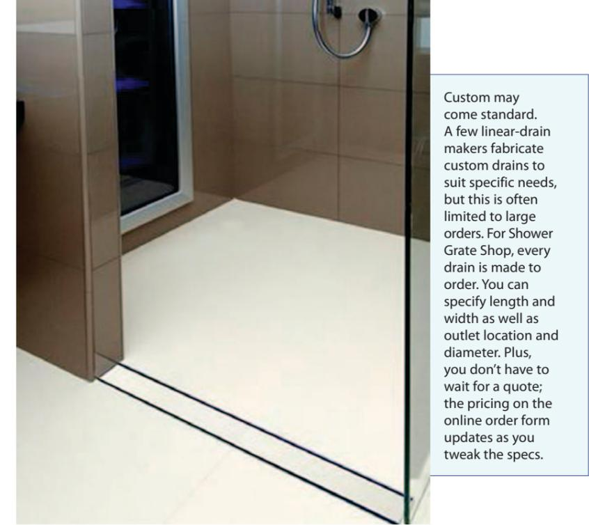
Custom may come standard. A few linear-drain makers fabricate custom drains to suit specific needs, but this is often limited to large orders. For Shower Grate Shop, every drain is made to order. You can specify length and width as well as outlet location and diameter. Plus, you don't have to wait for a quote; the pricing on the online order form updates as you tweak the specs.
