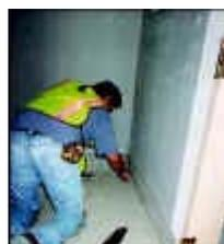
Some products used in composite sheets have definite limitations. For example, bituminous (peel and stick) waterproofing products can be susceptible to attack by the solvents used in stone sealers.
